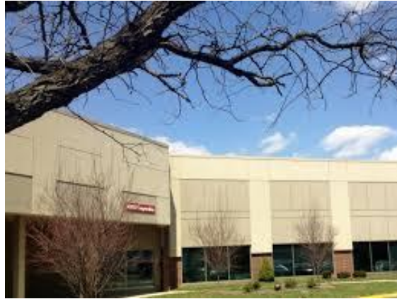
Headquarters in Mt. Laurel, New Jersey USA NYSE: INTT
