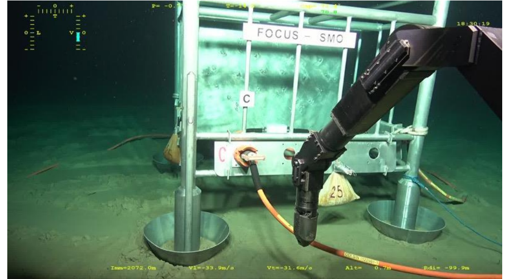
Connection to the Y junction box (using ROV Victor)
