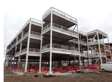
Steel & concrete frames
