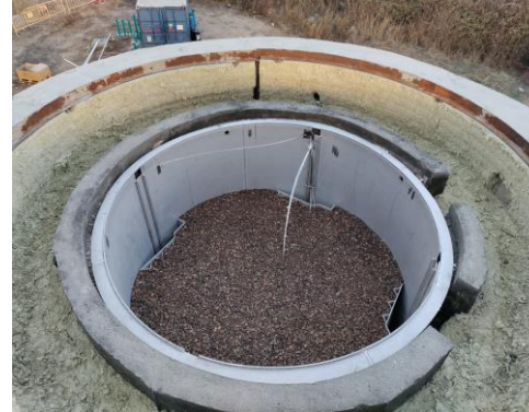
Temperature and strain monitoring in an energy storage concrete tank of a Concentrated Solar Power Plant
