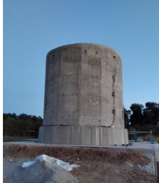
Temperature and strain monitoring in an energy storage concrete tank of a Concentrated Solar Power Plant
