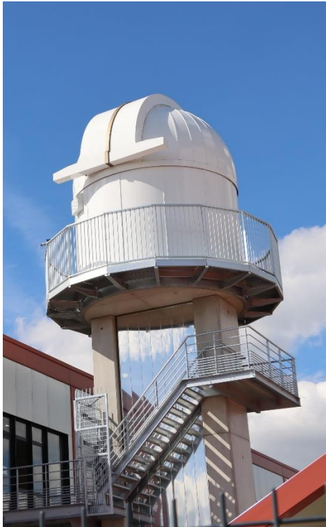
Operational optical Ground station
