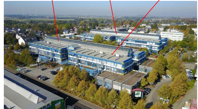
Technology Park Herzogenrath (TPH)
