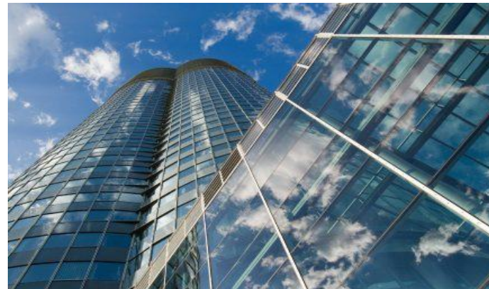
Facade with low-E glazing
