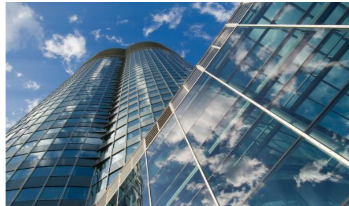
Facade with low-E glazing
