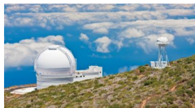
Ground station Field test
